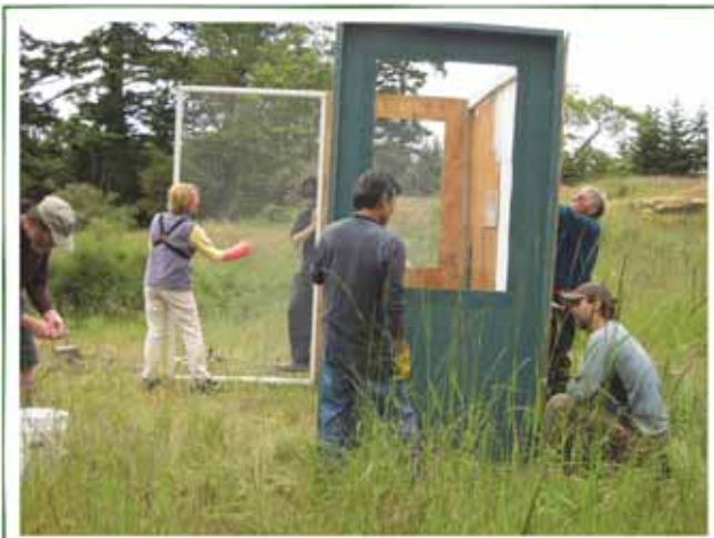
Constructing aviary © Gary Slater
